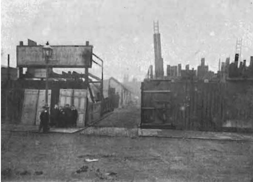
Figure 5. Closed to additional interments in the 1850s, the Peel Grove Burial Ground in Bethnal Green eventually became a storage yard for building supplies. Credit: Isabella M. Holmes, The London Burial Grounds: Notes on Their History from the Earliest Times to the Present Day (London: T. Fisher Unwin, 1896), 198.
